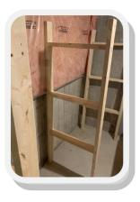
With helpers or bracing, stand the vertical support frames with the 20-inch clearance at the bottom.
