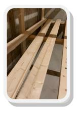
Starting from the bottom shelf, lay flat four 80-inch horizontal boards, perpendicular with the 24-inch width supports. Ensure the end of the 80-inch horizontal board is flush with the outside edge of the vertical support frames.
