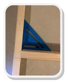
Use the carpenter square to align all boards, and attach the horizontal support to the vertical support with screws or nails.
