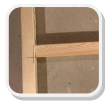
Position one of the 24-inch width dimension supports between and perpendicular to the 72-inch boards.
