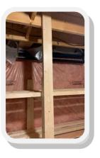
Use 3-Inch screws to fasten additional bracing to the workpiece and the celling joist.
