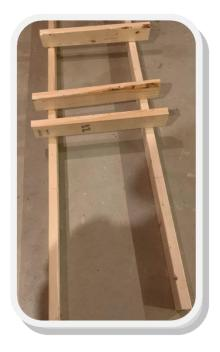
Lay two of the 72-inch vertical supports on the ground with the narrow faces positioned upwards.
