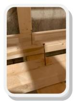
Fasten the 80-inch horizontal boards to the 24-inch width board with screws or nails.
